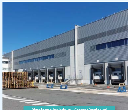
Plateforme logistique - Cestas (Bordeaux)
